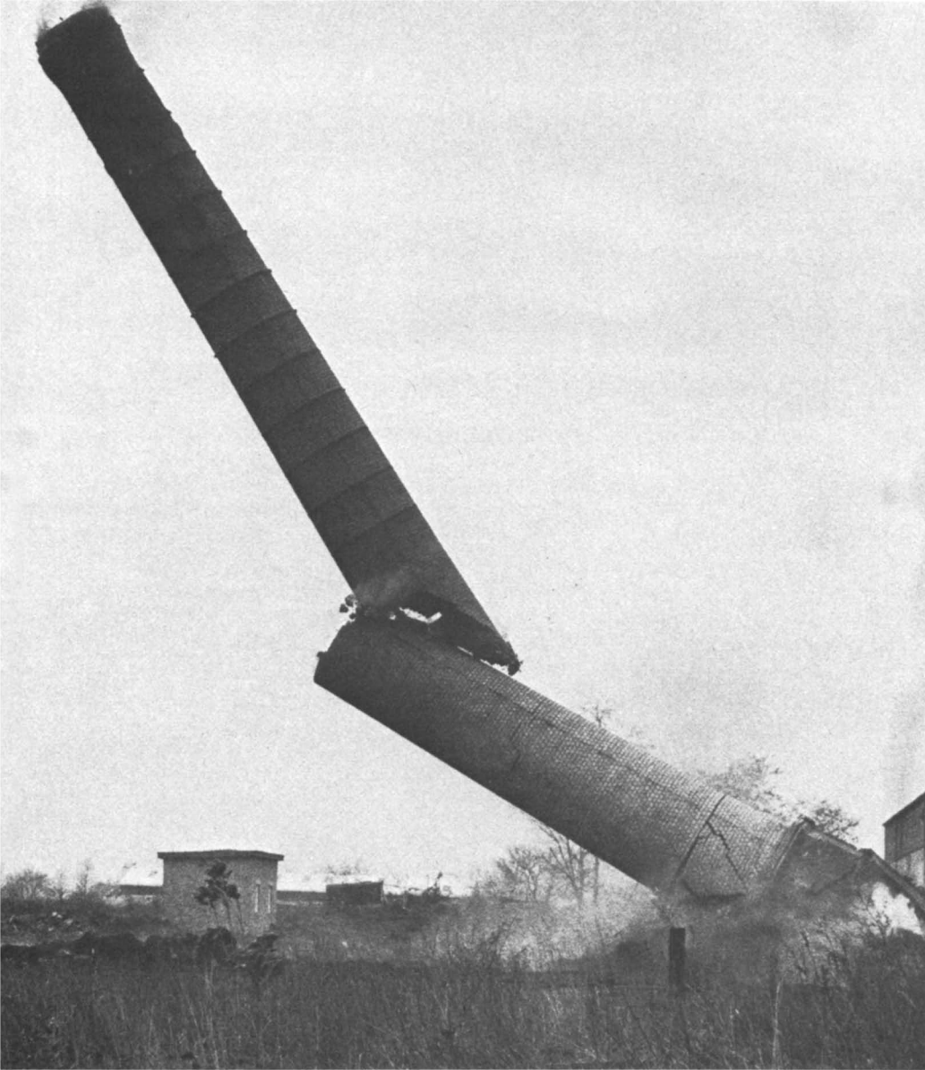
Fig. 2. The fall of a 49 m chimney in Louisville, KY. The major break is at approximately 0.47 h. Published with the permission of the Courier-Journal and Louisville Times .
